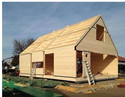
**Gambar 7.4** Rumah Modular Dengan Material CLT
