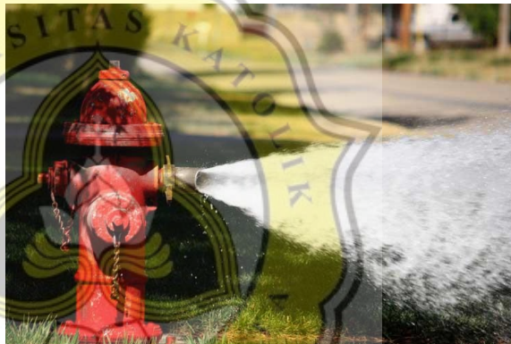
Gambar 7.21 Hydrant Pillar
