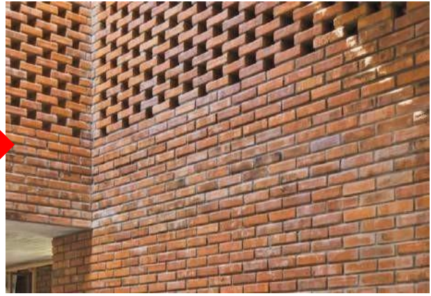
Gambar 5.7 Dinding Bata Expose
