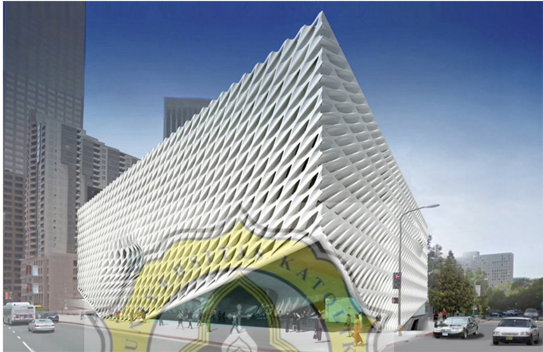
Picture 5.32 GFRC Facade Source: Thebroad.org
