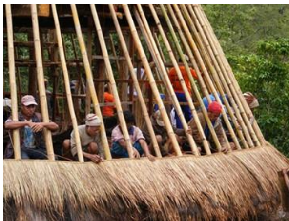
Gambar 3. Teknik Ikat rumbia/Rumbia for thatching/the art of lashing technique di Wae Rebo, Flores (Sumber: http://rahmanopick.blogspot.co.id/2015/02/wae-rebo-negeri-diatas-awan.html )
