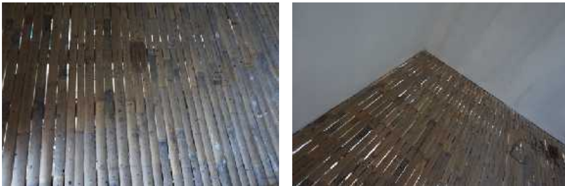
Figure 10 : the stage house's floor; preserved bamboo blades were used
