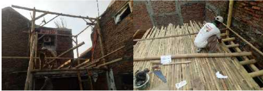
Figure 10: Installation of bamboo columns and floor (research documentation)
