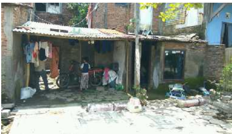
Figure 3: The house of Mr. Heri's family, the location of the hydraulic house construction with the material of Bamboo (research documentation)
