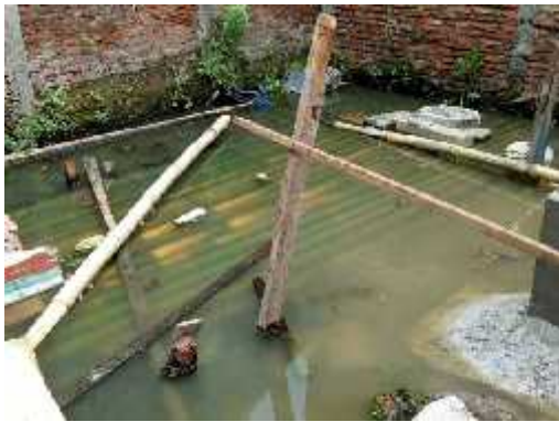
Figure 6: soaking part of the bamboo next to Mr. Heri's house (research documentation)
