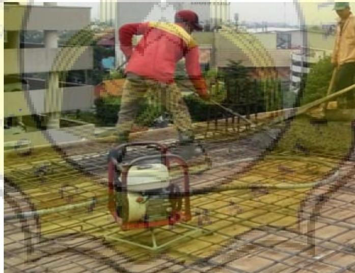
Gambar 3.29 *Concrete Vibrator*
