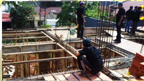
Gambar V-7 Atap Cor Dak Beton
