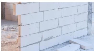
Gambar 56 Dinding Hebel
