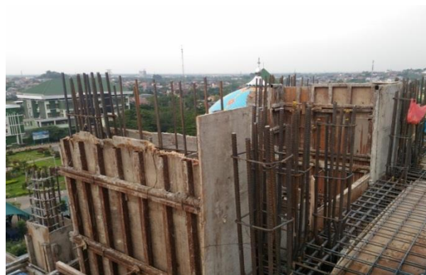
Gambar 3.25 Bekisting Core Wall
