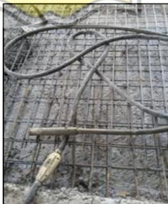
Gambar 3.46 Concrete vibrator
