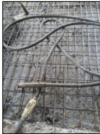
Gambar 3.45 Concrete Vibrator
