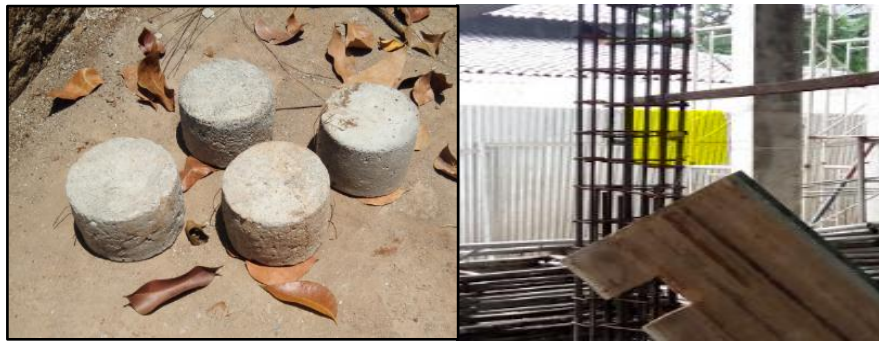
Gambar 3.56 Beton Decking
