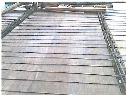
Gambar 3.21. bekisting plat lantai
