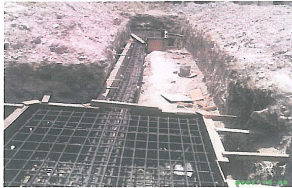
Gambar 3.11. Bekisting Tie Beam
