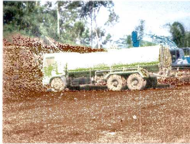
Gambar 3. 31 Water Tank Truck (Sumber: Dokumentasi Pribadi)
