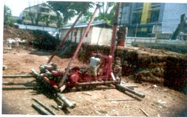
Gambar 5.3: Alat pancang hammer
