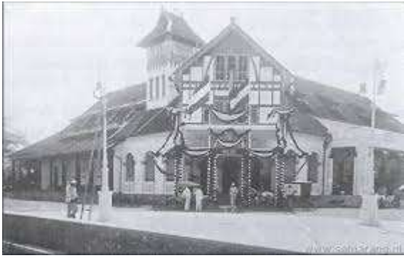
Figure 4 The old GRIS heritage building that has been demolished
