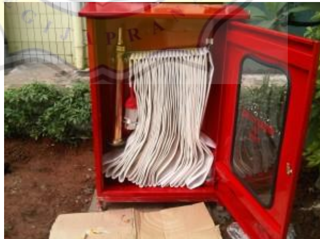
Gambar 3. 37 Hydrant Box Sumber: allaboutsafety.co.id
