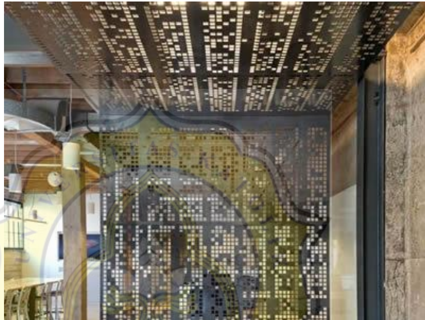
Gambar 3. 30 Material Plafon Jenis Perforated Metal Sumber: perforated-plate.com
