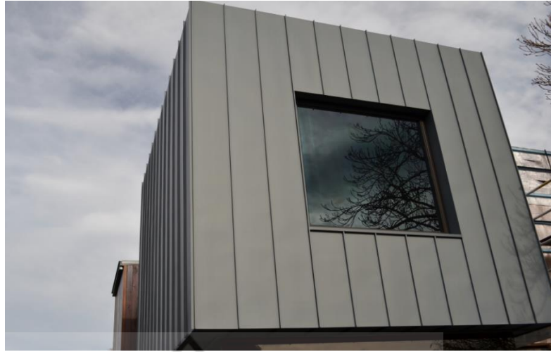
Gambar 3. 32 Zinc Roof Cladding Sumber: roofglaze.co.uk
