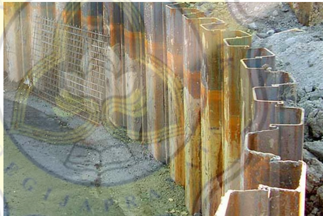
Gambar 3. 17 Retaining Wall Jenis Sheet Pile Sumber: civilengineersforum.com
