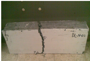
Figure 6. The crack pattern of confined beam of specimen BL-N-03 (Photograph by Setyanegara and Sagita, 2008)
