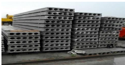
Gambar 3. 38 Pelat Pre Cast Hollow
