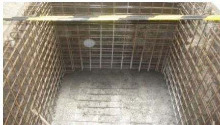
Gambar 3. 41 Dinding masive beton (google.com)
