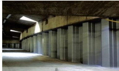
Gambar 3. 33 Dinding Penahan Tanah Sheet Pile (google.com)
