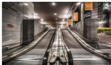
Gambar 3. 71 Ramp Escalator (google.com)
