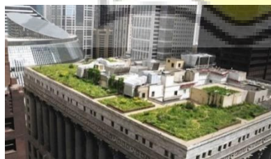
Gambar 3. 55 Roof Garden (google.com)
