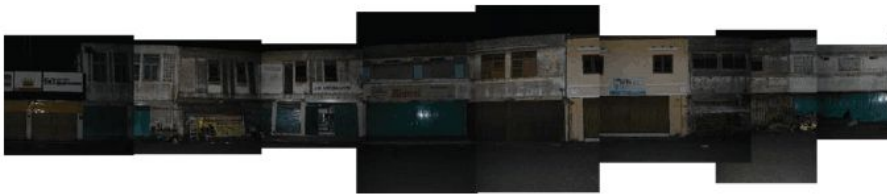
Figure 3 Pekojan street at night
