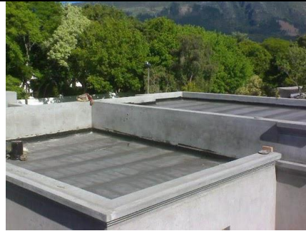
Gambar 3 12 Atap dak beton Sumber: rizkifachurohman.blogspot.co.id
