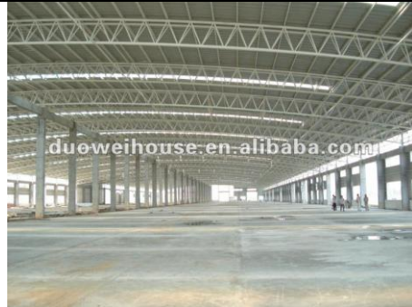
Gambar 3 10 Space truss Sumber: duoweihouse.alibaba.com
