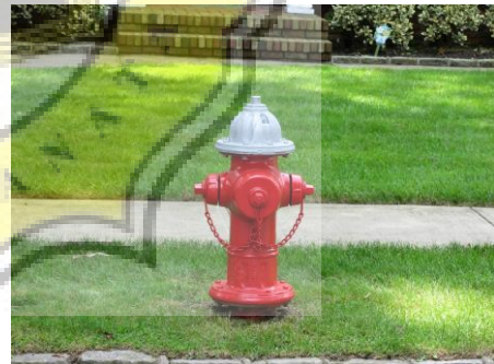
Gambar 3 34 Hydrant taman Sumber: gcpwater.org
