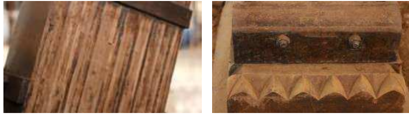
Gambar 5.1.2.C Detail Laminated Wood dan Pemberat Besi (Sumber : RESTORATION PROJECT - BARAKGEBOUW A)
