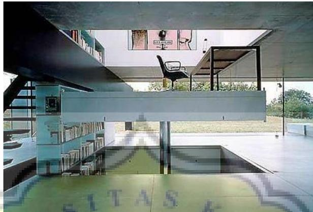
Gambar 3. 8 Contoh sistem *moveable floor*
