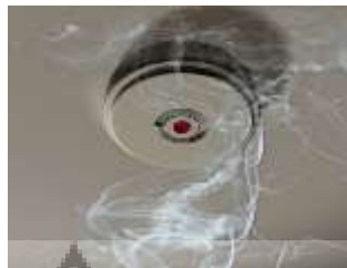
Gambar 3.2.2.1 Smoke Detector
