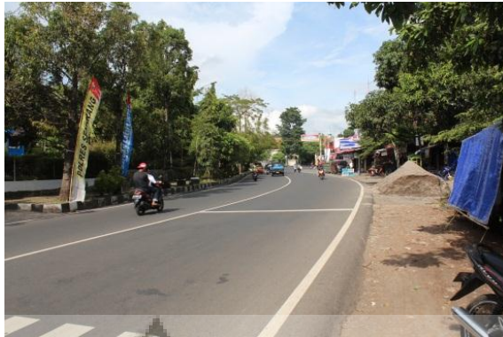
Gambar 103. Jalan Mgr. Sugiyapranata
