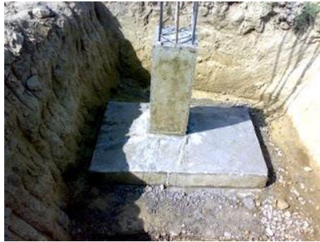
Gambar 53. Pondasi Footplate
