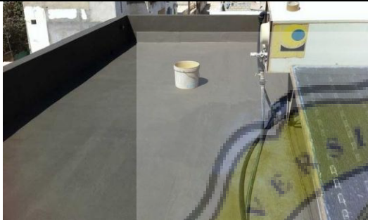
Gambar 45. Dak Beton Sumber: 3.bp.blogspot.com
