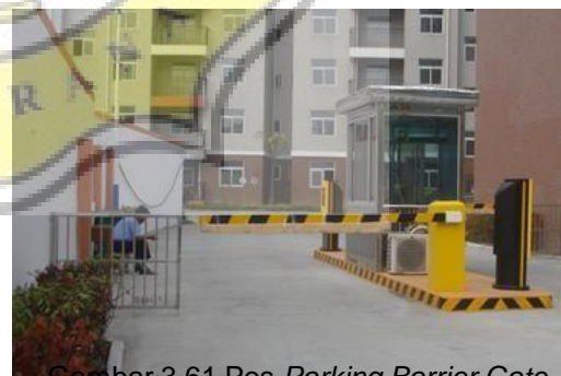
Gambar 3.61 Pos Parking Barrier Gate
