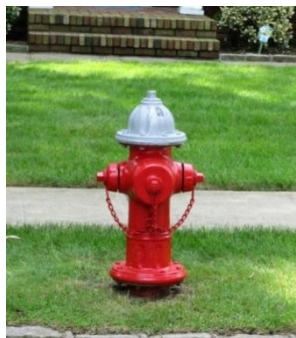
Gambar 3.33 : Kotak Hydrant, Pole Hydrant, Fire Hydrant
