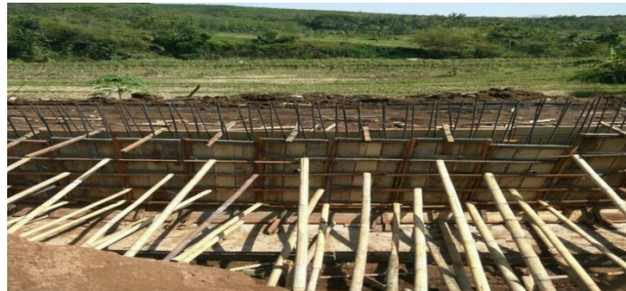
Gambar 3. 1. Bekisting Dinding Penahan Tanah
