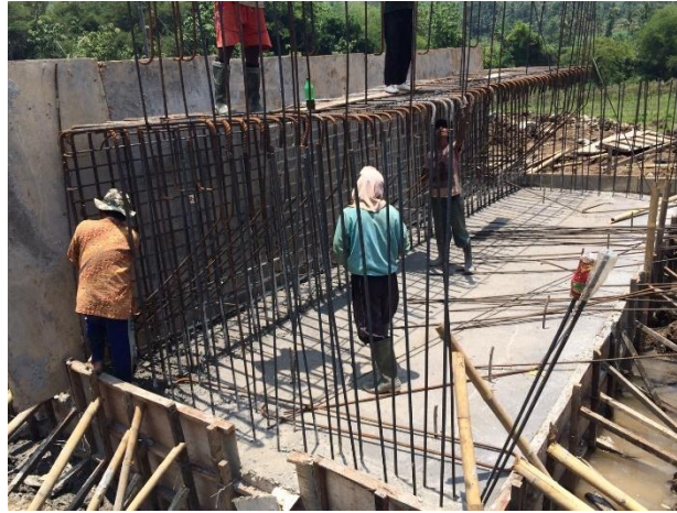
Gambar 3. 3. Pembesian Abutment
