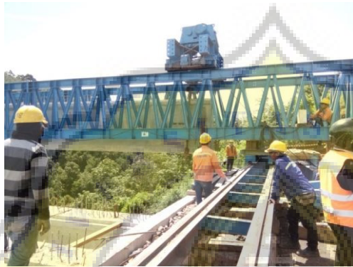
Gambar 3.46 Launching Girder
