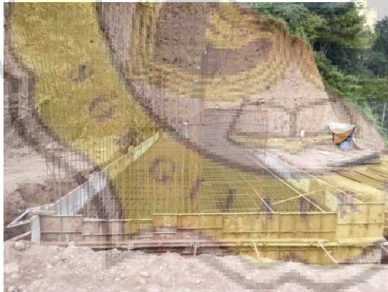
Gambar 3.10 Penulangan Abutment 1
