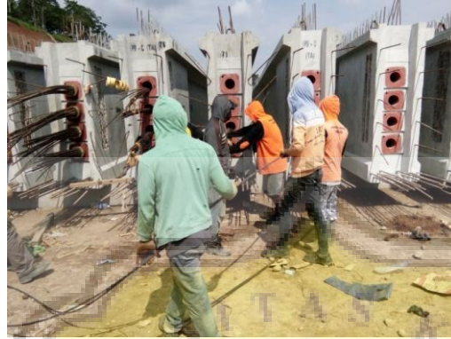
Gambar 3.19 Proses Grouting
