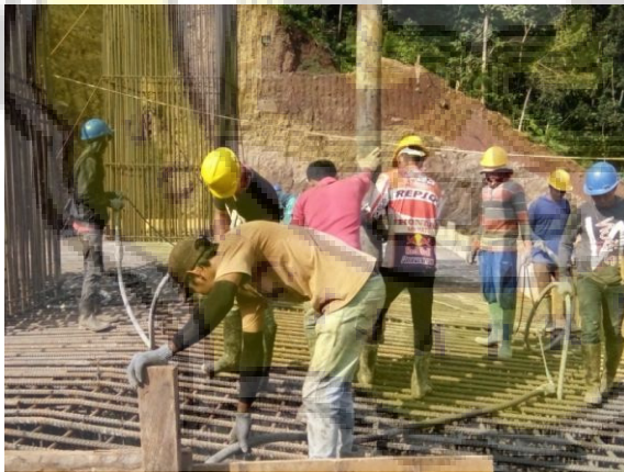
Gambar 3.8 Pengecoran Footing
