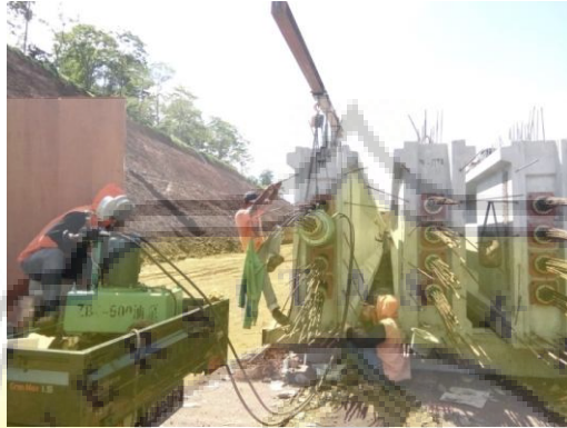
Gambar 3.17 Proses Stressing
