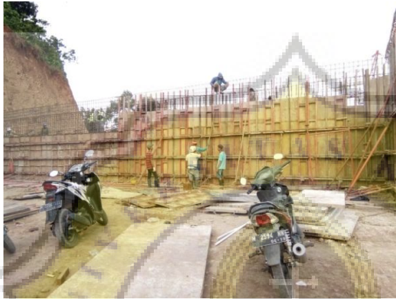
Gambar 3.11 Pemasangan Bekisting Abutment 1
