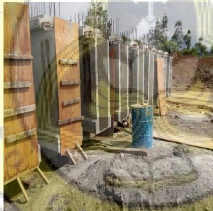
Gambar 3.20 Hasil Proses Stressing dan Grouting
