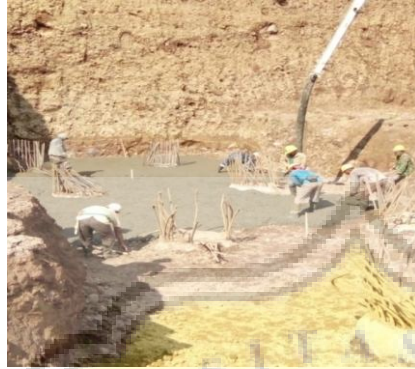
Gambar 3.9 Pengecoran Footing
