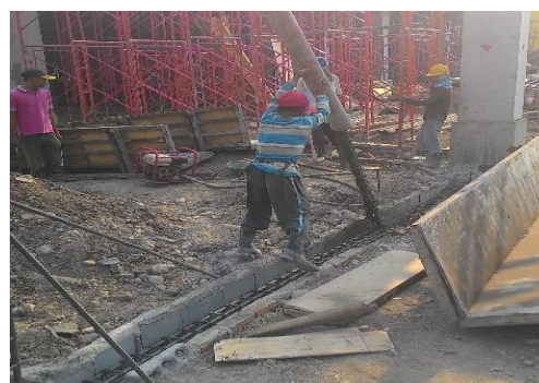
Gambar 3.8 Pengecoran Tie Beam
