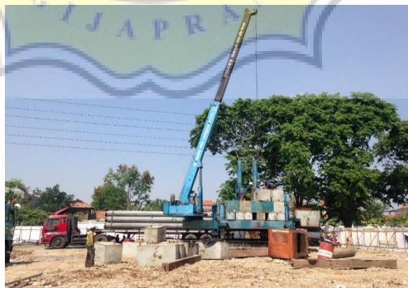
Gambar 3.2 Alat Hydraulic Static Pile Driver (HSPD)
