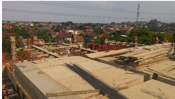
Gambar 3.14 Bekisting Plat Lantai
