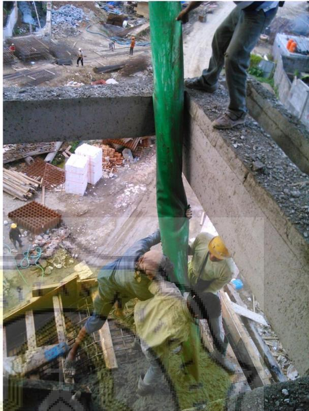
**Gambar 3.31 Tremi *Concrete Bucket***
