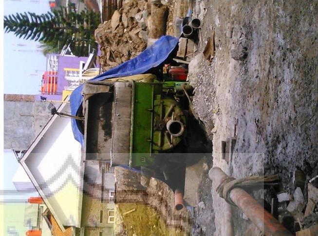
**Gambar 3.21 Concrete Pump**
