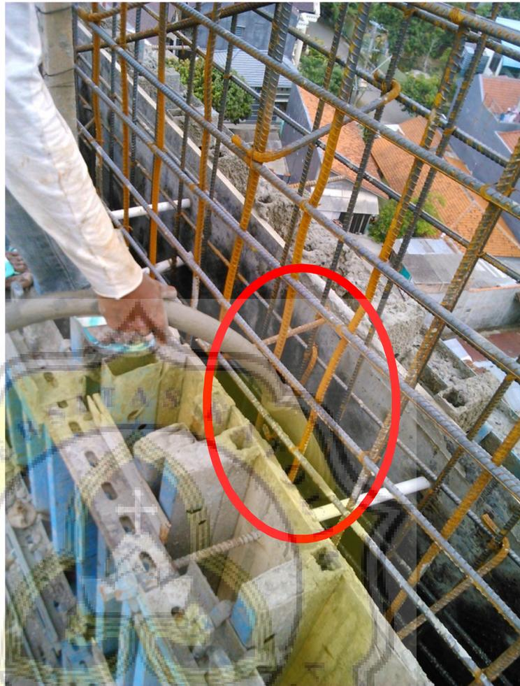
**Gambar 3.27 Concrete Vibrator**
