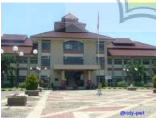
Gambar 5.90 Gedung Terminal Purwokerto
